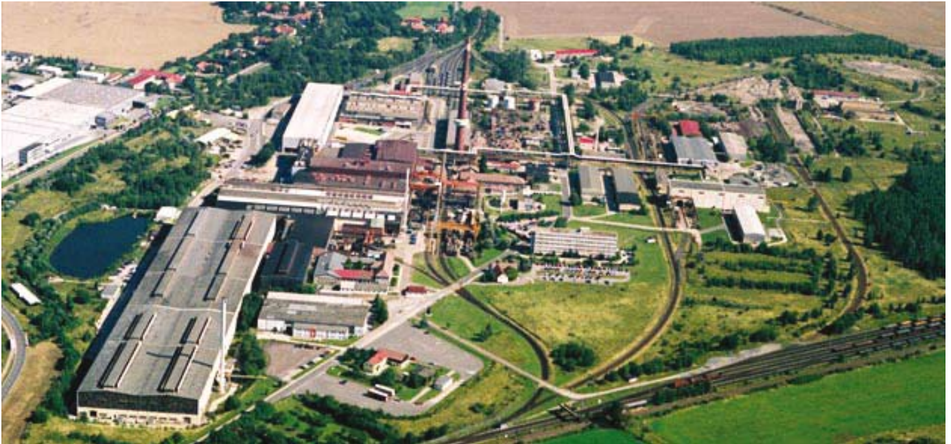
Plant grounds of Ilsenburger Grobblech GmbH
