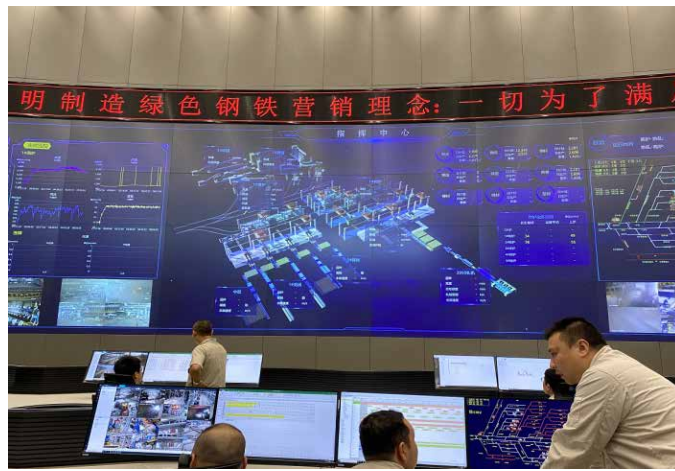
Control room at HBIS TangSteel New District.
