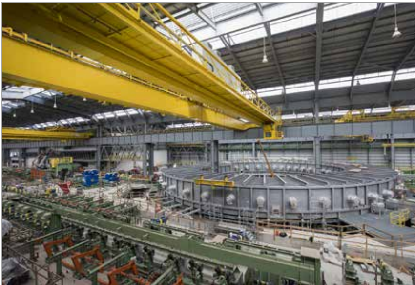
Bau des Drehofens in TenarisBayCity.
