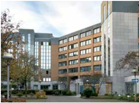
The new office building of PSI Metals Head Office in Düsseldorf.
